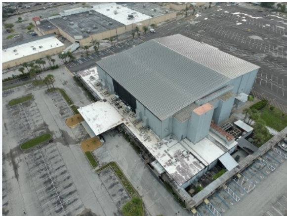
IMAGE 03 Oblique view of main and low-slope roof areas
