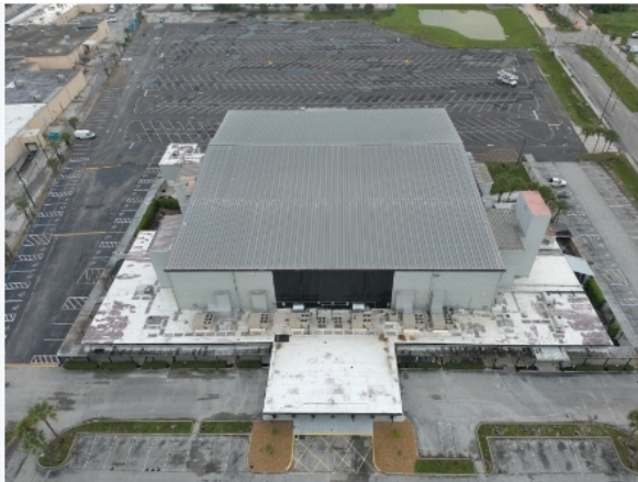
IMAGE 01 Front overview and perimeter roof systems
