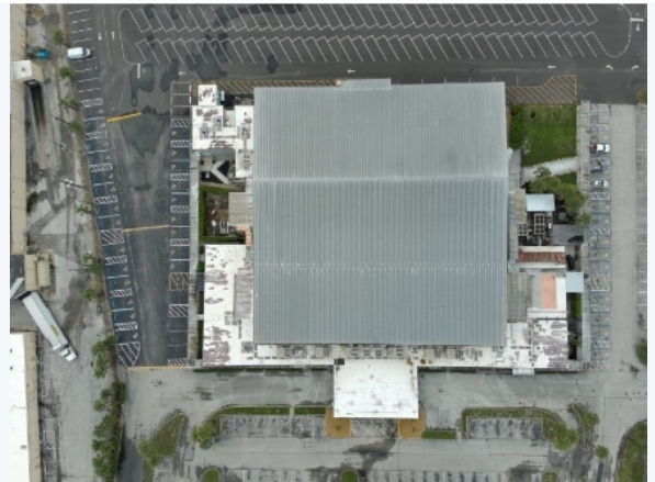
IMAGE 02 Nadir overview of the full roof layout
